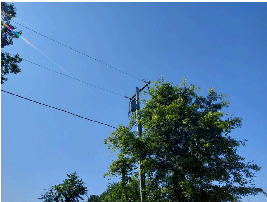
Photo 40 : On-site pole mounted transformer.
